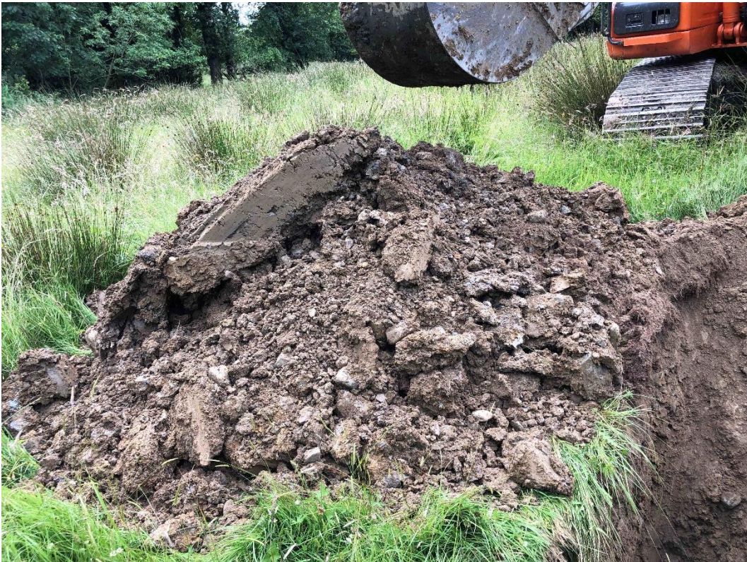
Photo No. 14 – Trial Pit 6 Arrisings
