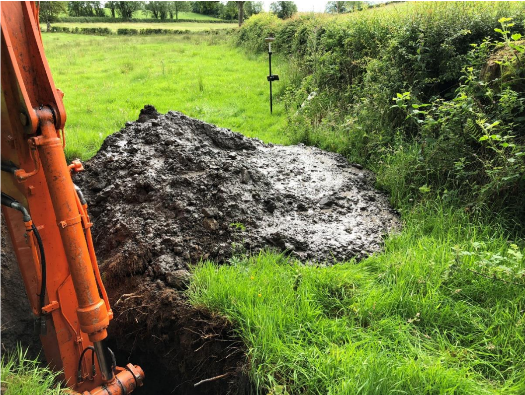
Photo No. 1 – Trial Pit 1 Arrisings
