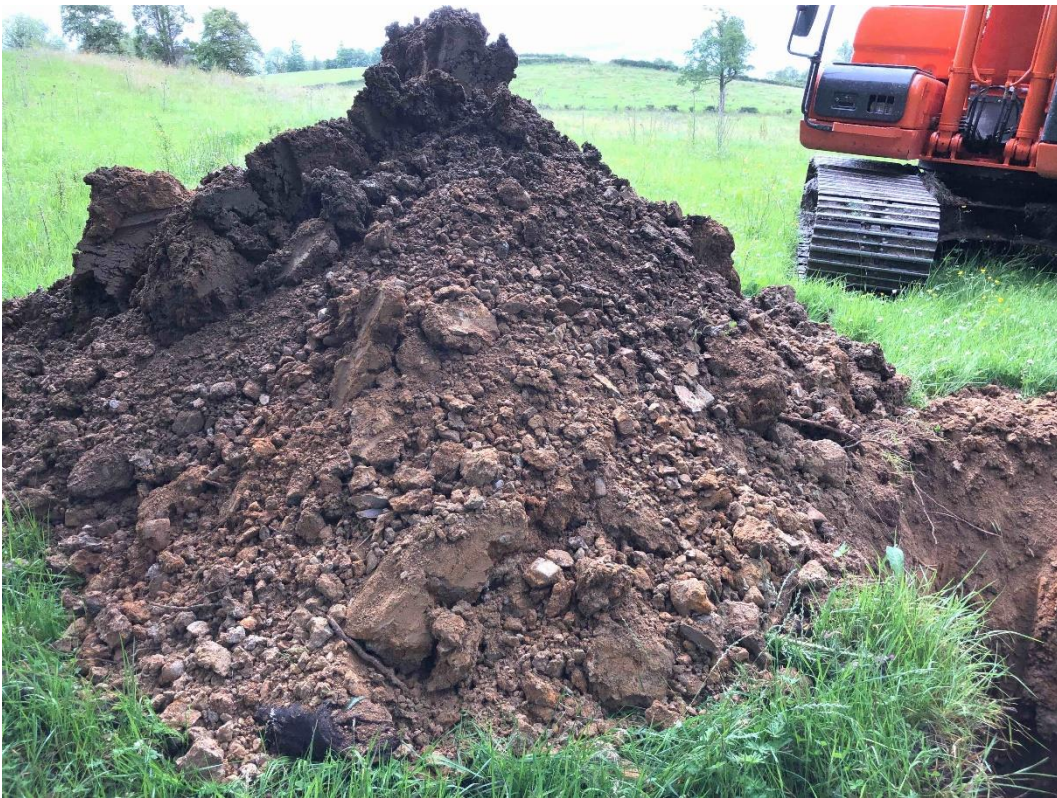
Photo No. 4 – Trial Pit 2 Arrisings
