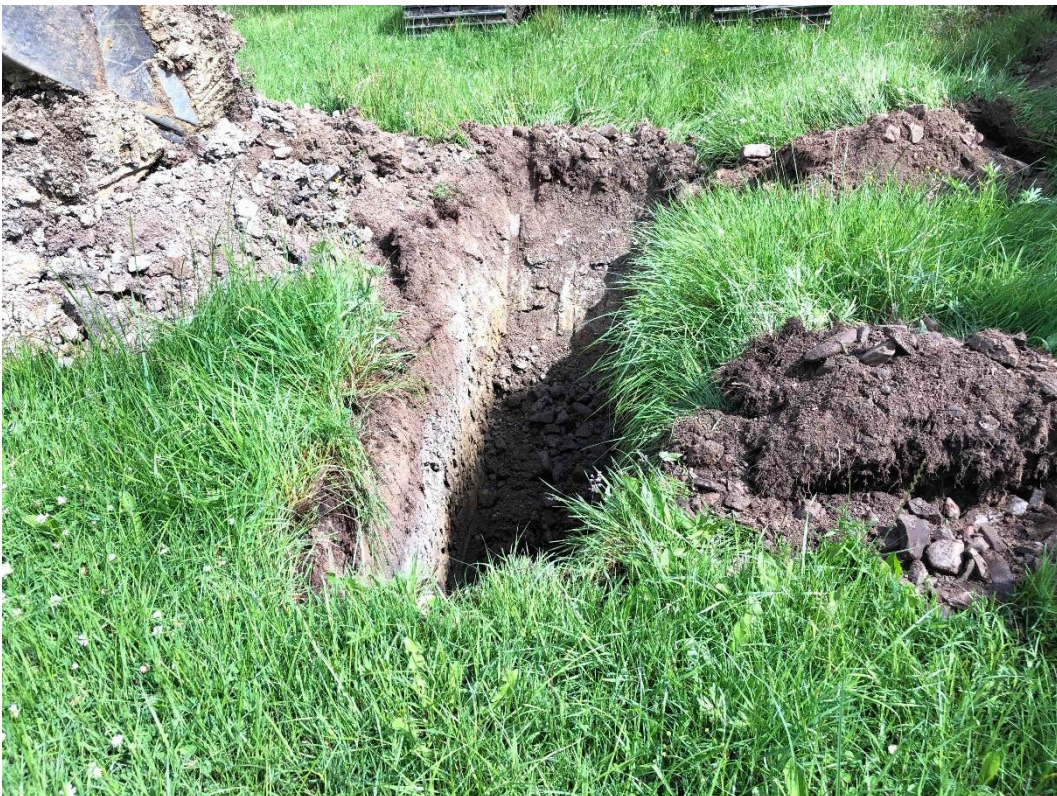
Photo No. 6 – Trial Pit 3 Arrisings
