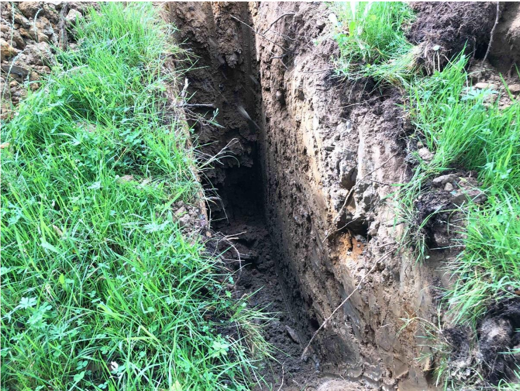
Photo No. 2 – Trial Pit 2
