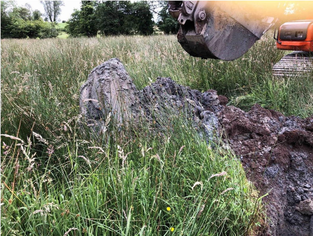
Photo No. 11 – Trial Pit 5 Arrisings
